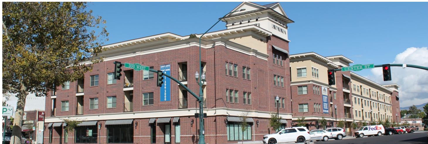
Liberty Center completed on 300 West between Center and 100 North
