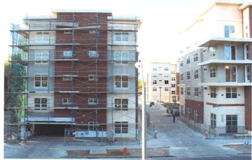
Pictured above, the Temple View Apartments under construction.
