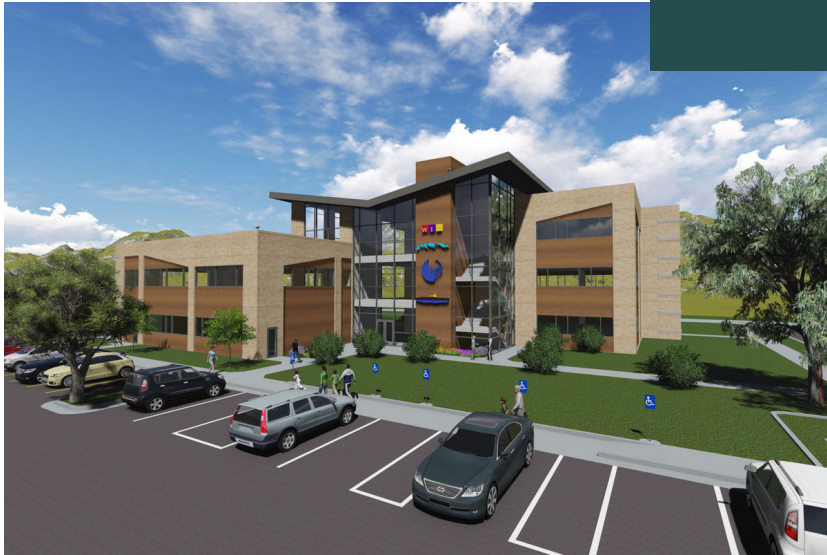
Facilitated the construction of the new Wasatch Mental Health facility in Payson
